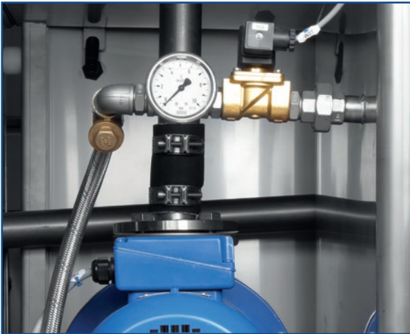
Manometer for pressure checks - simple functional control
