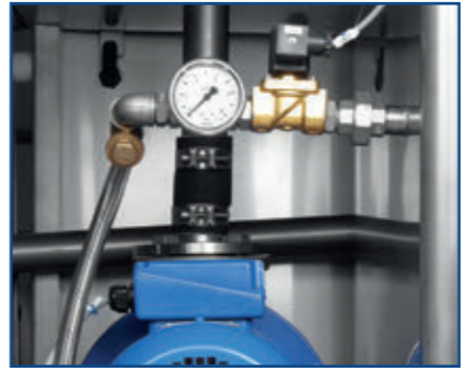
Image 18 Pressure gauge for pressure testing - simple function check
